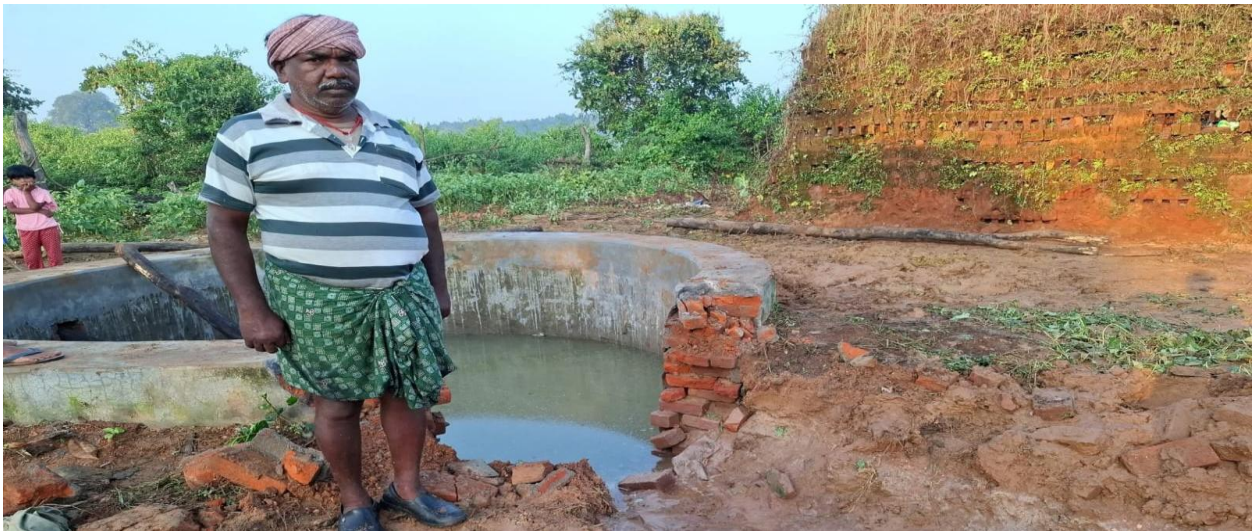
Figure 8. A local resident stands beside the partially damaged open well in Khaira Village, Jharkhand, where the 7-day-old elephant calf accidentally fell on 15 October 2025. The photograph, captured after the rescue operation, highlights the structural vulnerability of such wells and the urgent need for preventive measures to reduce wildlife accidents in elephant-movement zones.
